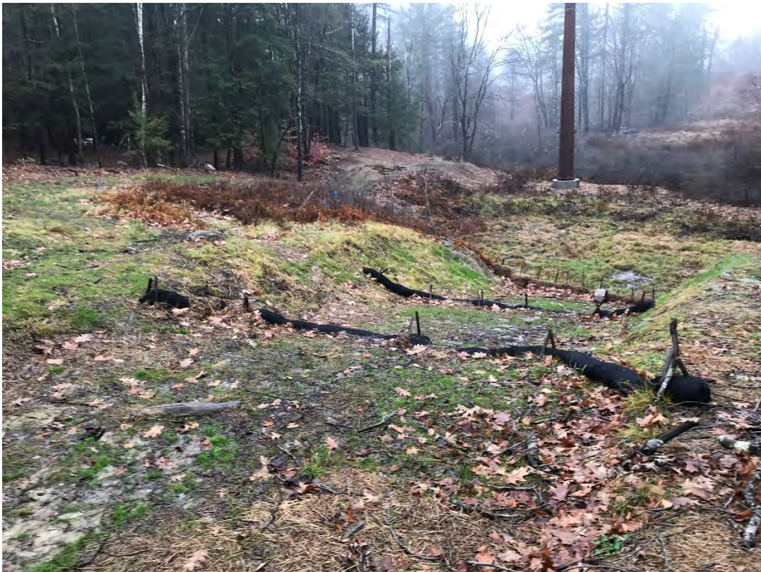
Fig 10: Slope between Strs. 28 and 29. Viewing north. (12-01-20)
