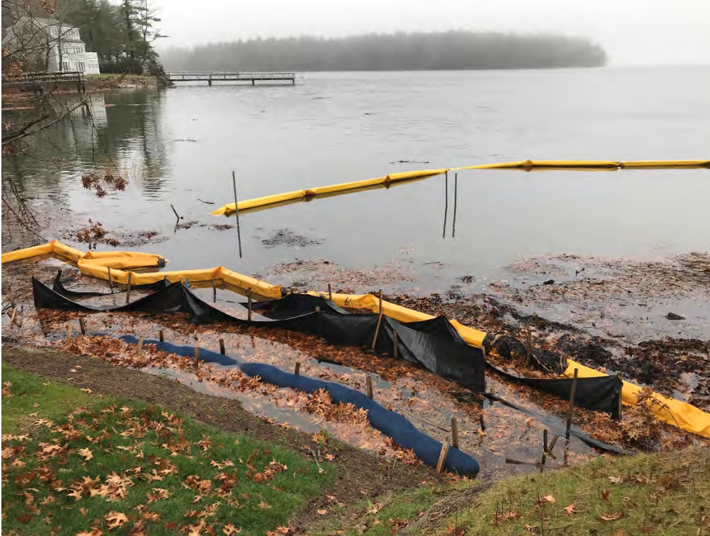
Fig 5: Toe of the slope at Gundalow Landing/east side of the bay. Viewing south. (12-01-20)
