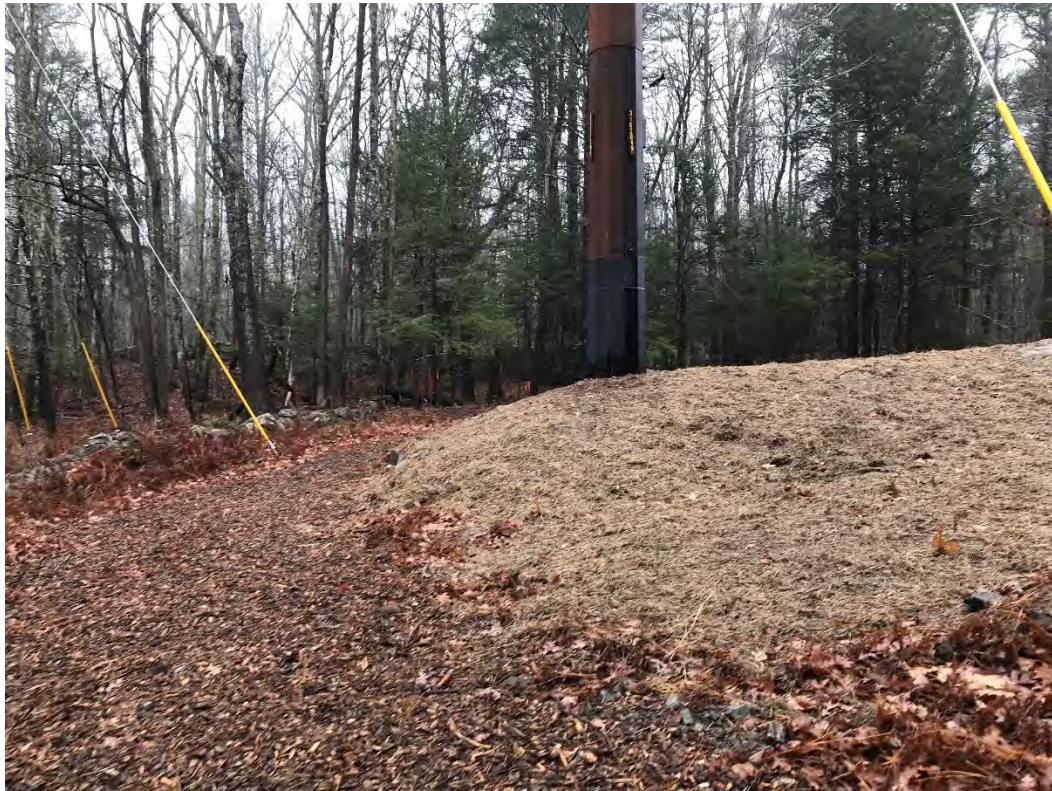
Fig 8: Str. 90 work area. Viewing southwest. (12-01-20)
