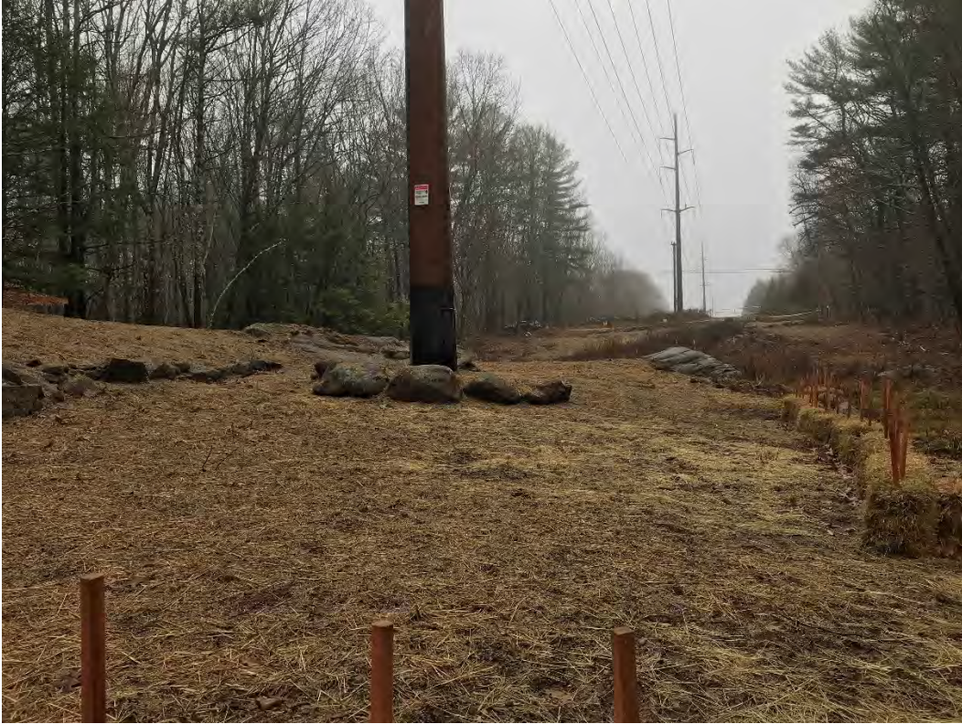
Fig 7: Str. 89 work area. Viewing northwest. (12-01-20)
